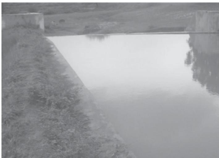
**Fig. 5.** Concrete check dam across the creek in watershed area, Hazaribagh, Source: Singh *et al.* (2006)
